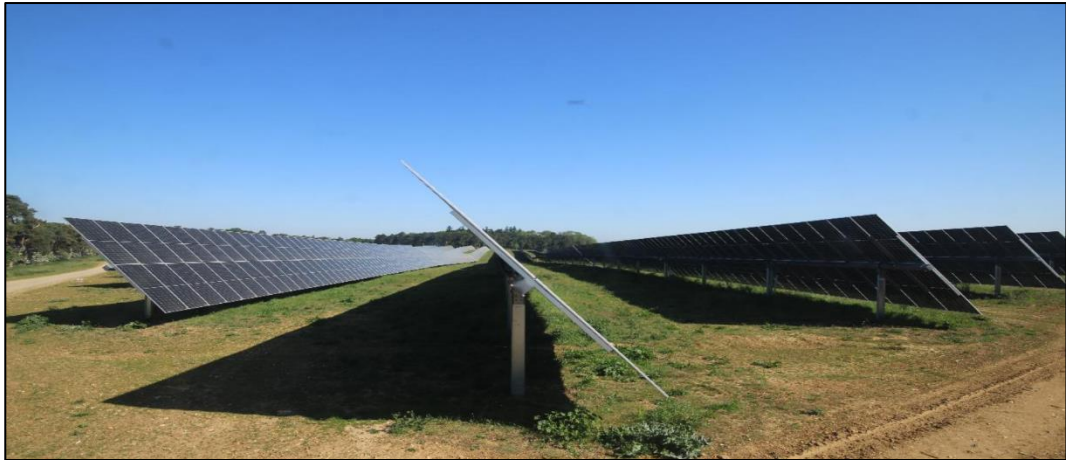
Plate 3-2: Typical Tracker Solar PV Panels in a Near Flat Orientation
