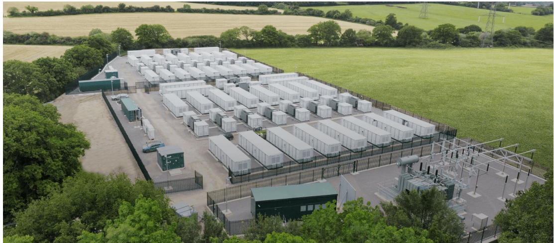
Plate 3-9: Typical Battery Energy Storage System
