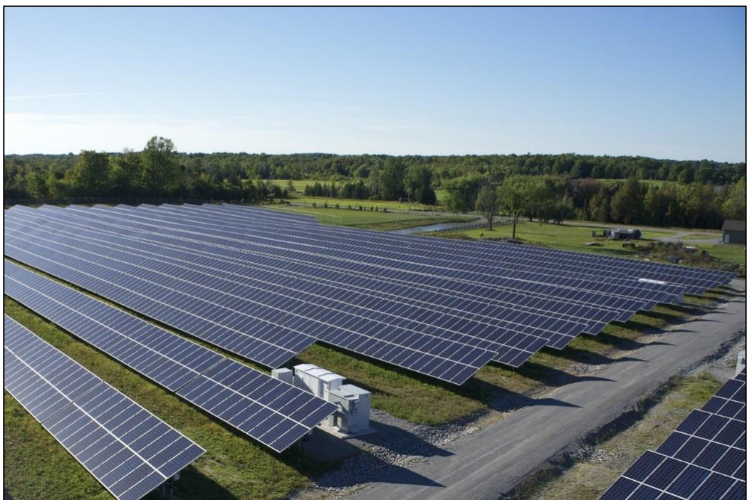
Plate 3-5: Typical Fixed Solar PV Panels (with Conversion Unit/Inverter)
