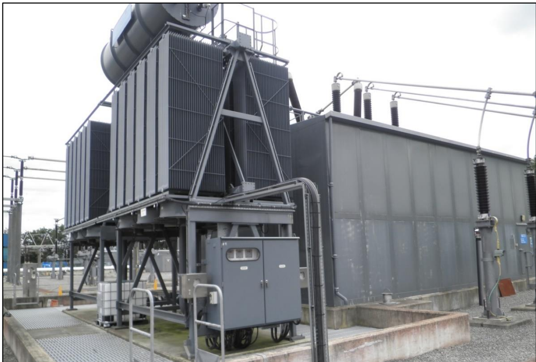
Plate 3-11: Typical (Large 400 kV) Power Transformer
