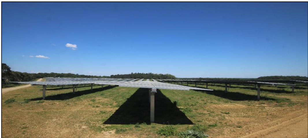
Plate 3-3: Illustration Tracker Solar PV Panels following the sun position
